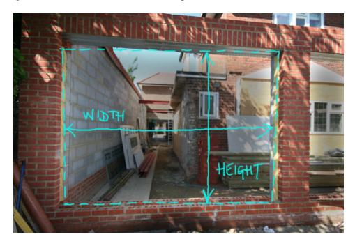
If the height dimensions on either side of the opening are the same and the width dimensions at the top and bottom are also the same, then the two diagonals must be identical. This is the easiest way to check the dimensions are correct.
